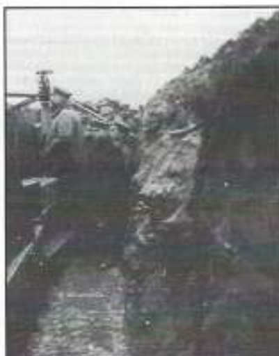
German surveyors in the trenches 1916.
