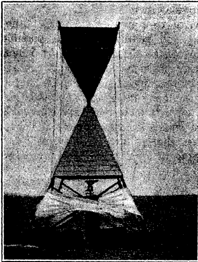
IRON QUADRIPOD BEACON, WITH WOODEN BATTENS.
