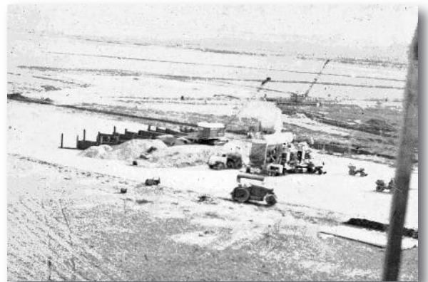
Catfoss site during construction taken from Catfoss tower.
