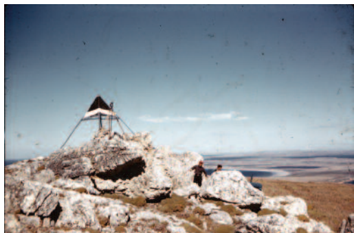
Beacon being erected on First Mt., Pebble Island 10 Jan 1958.
