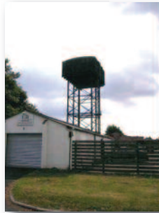
Typical water tower trig point on top,
