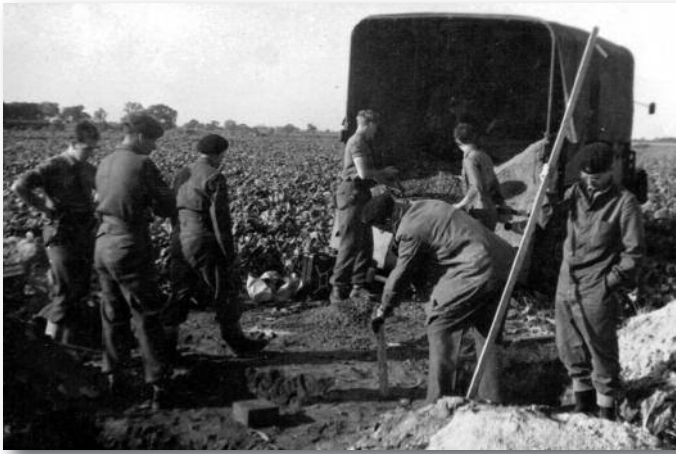
This picture shows pillar building ready to centre the surface mark.
