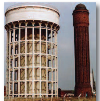
Goole Water Tower, trig point on top used during Driffield complex.
