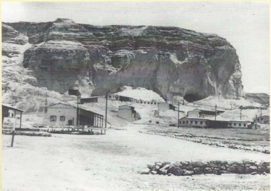
The camp at Tura and the entrances to the caves where 512 Field Survey Company produced the faked map.
